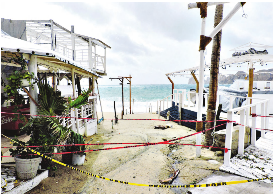
▲ Caution tapes prevent the passage at El Medano beach, as Hurricane Hilary hits Mexico's Baja California peninsula, in Cabo San Lucas, Mexico.
