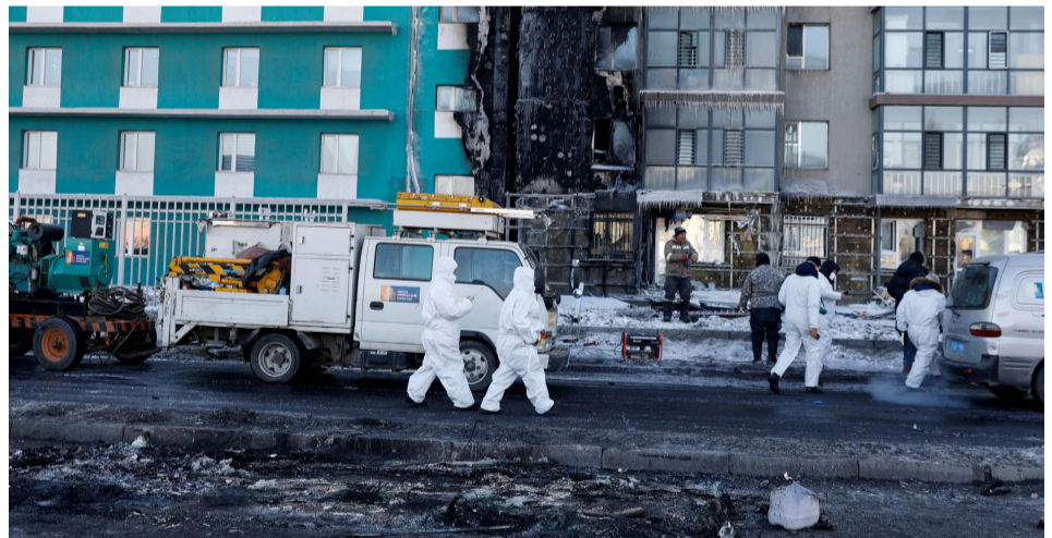
▲ Experts in PPE walk to a building damaged by an explosion after a truck carrying liquefied natural gas crashed, in Ulaanbaatar, Mongolia.
