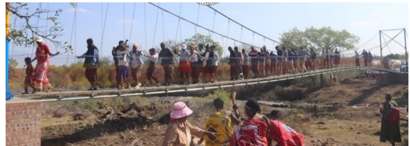
▲ New Ngobojaneni suspension footbridge.
